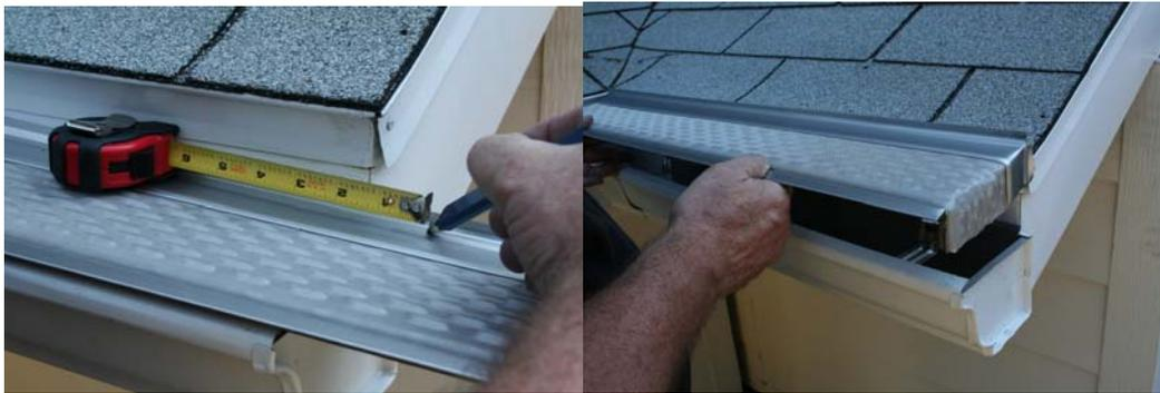
**Step 4,** Optional screws may be utilized at the sight line channel into the fascia to provide additional structural support for the entire gutter system.
