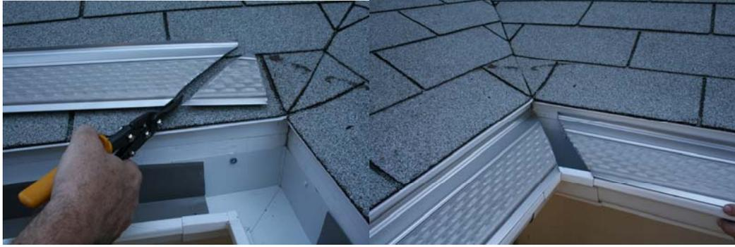
**Step 3.** At the termination end of the gutter system, you will need to snip and remove the panel nose and the weep hole leg approximately 2" from the gutter end. Bend the 2" section downward at a 90 degree angle to create a cap at the end of the system. This will prevent debris and pest from entering the gutter system at the end
