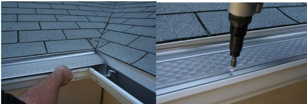
**Step 2.** When reaching the gutter corner, mark and cut a diagonal angle beginning from the gutter nose. Begin the **Clean-Mesh** panel angle cut at the front lip, then snip the weep hole leg, and begin the angle cut at the gutter systems back corner and cut towards the front of the panel. Cut and remove the face of the next **Clean-Mesh** panel to conform to the angle and butt tight together.
